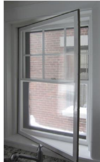
Insert being installed
